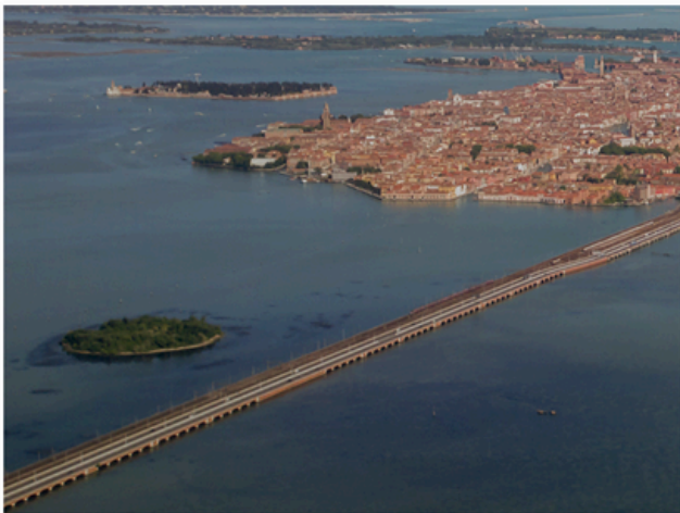
Libertà Bridge over Venice Lagoon, the longest Italian bridge (3'850 m)
